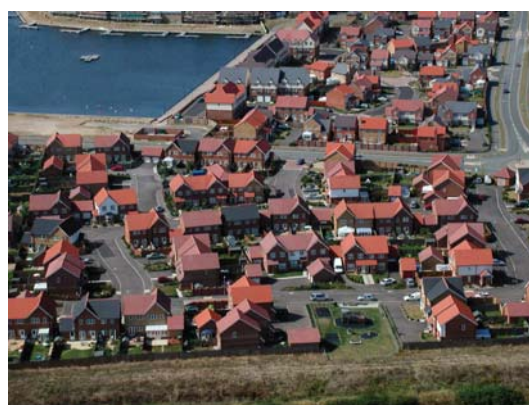
Housing Development in Sovereign Harbour
