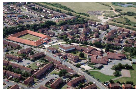
Shinewater Community Centre
